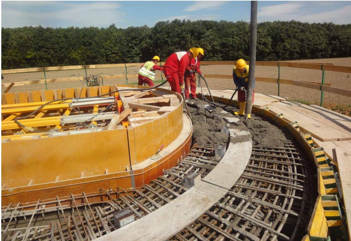
**Abbildung 1: Betonage Fundament / concreting foundation**
